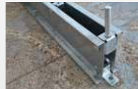
The racking is fixed to the floor using M10 x 90mm anchor bolts.
