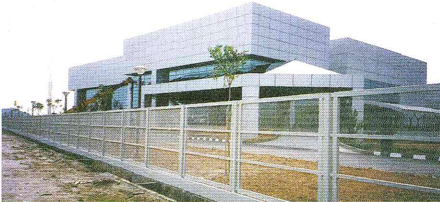
Expanded Metal Fencing
